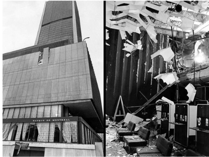
One of the most spectacular actions of the Front de libération du Québec (FLQ) involved the explosion of a bomb at the Montréal Stock Exchange in 1969. The photos show the damage caused by the explosion outdoors and inside the building. La Presse , February 4th, 1969, p. 7.
